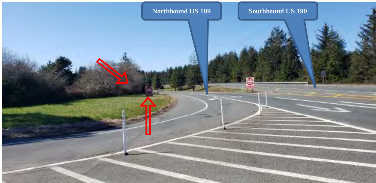
Figure 1: February 27th, 2020-EVCR looking at approaching north bound US 199 traffic
